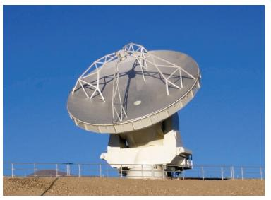
Figure 2: An ALMA antenna showing the main reflector, subreflector and central hole.
