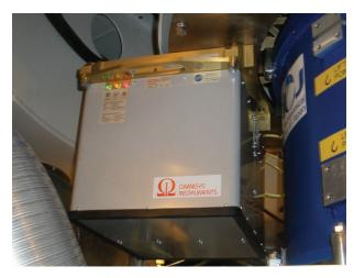
Figure 4. A water vapour radiometer installed in the receiver cabin.
