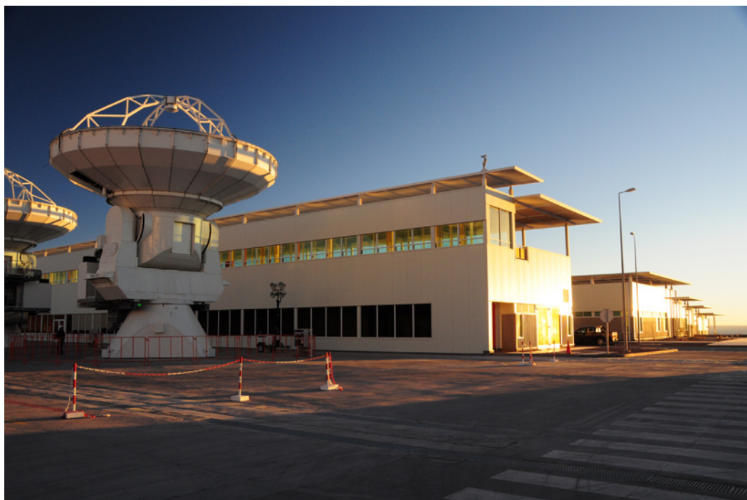
The OSF Technical Facility and two antennas at sunset
