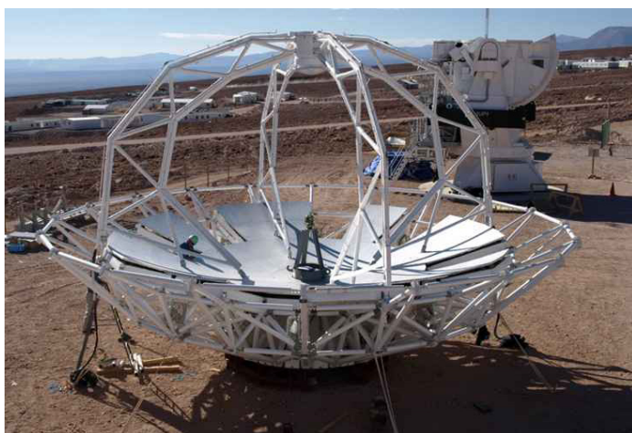
ALMA has reserved large areas in the OSF for the assembly work by the antenna vendors. These are the Site Erection Facilities (SEF). MELCO, having performed almost complete erection in Japan, has decided not to use any building for the final integration on site. Shown here is the mounting of the panels for the main reflector on the backup structure.
