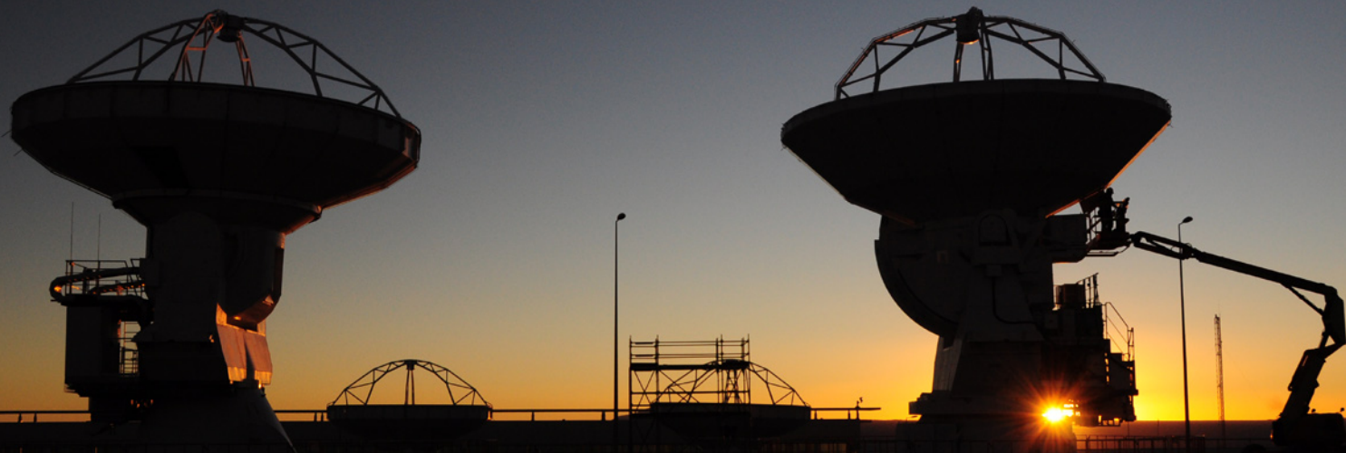
A view from the upper level of the OSF antenna area at the sunset, showing MELCO antenna #3 on the left, and Vertex antenna #2 on the right. In the background, the top of OSF TF and the topmost structure of two Vertex antennas can be seen.
