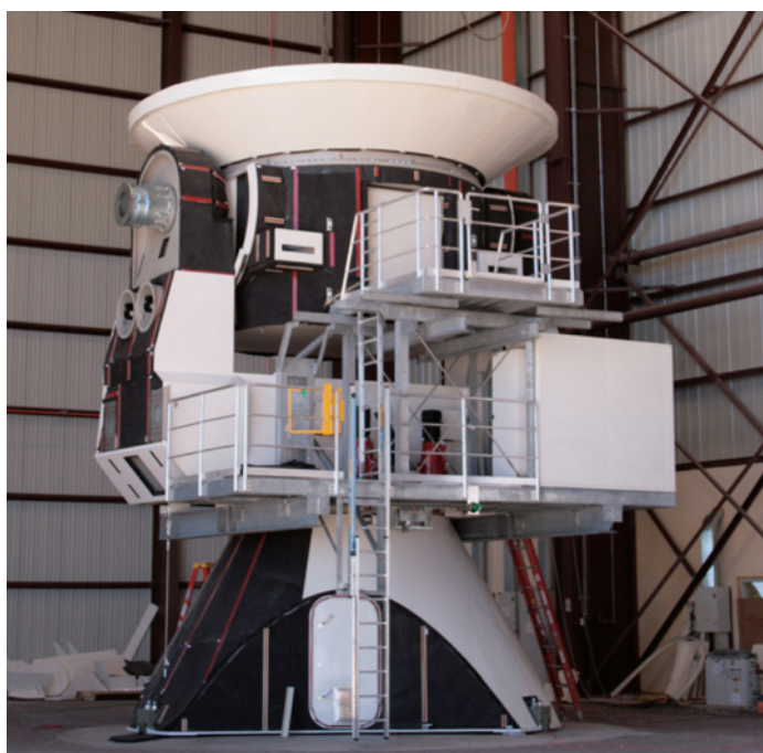
ALMA has reserved large areas in the OSF for the assembly work by the antenna vendors. These are the Site Erection Facilities (SEF). MELCO, having performed almost complete erection in Japan, has decided not to use any building for the final integration on site. Shown here is the mounting of the panels for the main reflector on the backup structure.
