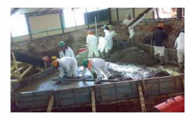
3. A later stage of the pouring. The lean concrete (shown being poured at the back of this picture) is being leveled. The station is covered to provide a higher temperature while the concrete hardens, the so-called curing process. The red cylinder in the lower right is a heater used to provide warmth during the concrete curing process. During the entire time, the temperature is constantly monitored.
