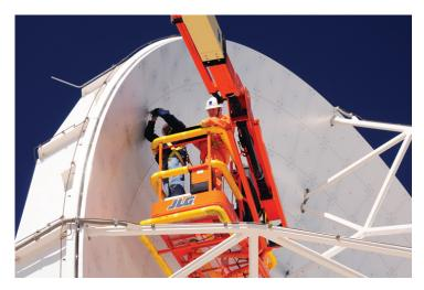
Holography campaign: panels adjustment on an antenna
