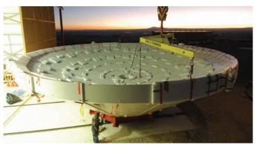
This photo was taken at the OSF. The 1st backup structure covered with protective foams is mounted on the integration jig foreseen for panel integration, prior to be moved inside the European Antenna Consortium BUS integration building.
