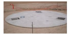
6. Station after the concrete work was finished. The next steps are to mount inserts in the three openings. These inserts will ensure that the antenna is accurately placed on the station and also provide a strong and solid connection between station and antenna. The two covered openings are for the power and signal transmission vaults.
