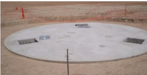
6. Station after the concrete work was finished. The next steps are to mount inserts in the three openings. These inserts will ensure that the antenna is accurately placed on the station and also provide a strong and solid connection between station and antenna. The two covered openings are for the power and signal transmission vaults.
