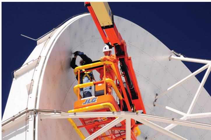
*Holography campaign: panels adjustment on an antenna*
