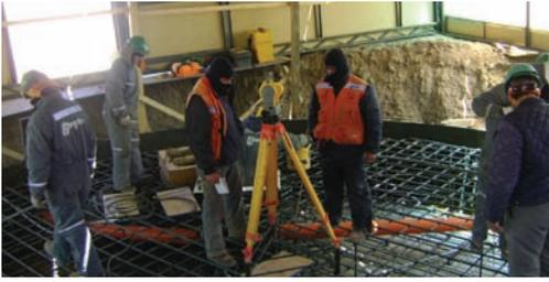
4. Preparations for pouring the upper level of concrete. This is to be denser structural concrete (type G-250) with a reinforcing cage (lean concrete does not require this cage). The red tube in the middle of the station is a conduit for signal and power cables. The level is used to ensure that the construction is as close to horizontal as possible.
