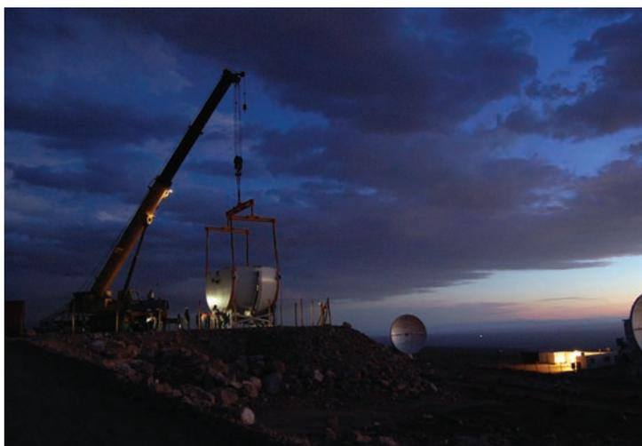
*The preliminary steps for assembly of the European Antenna Consortium antennas at the Site Erection Facility (SEF). In this view, a crane is lifting the lower part of the antenna, containing the elevation drive system. The SEFs for each antenna supplier are located close to but below the OSF building. On the right are two Mitsubishi Electric Company (MELCO) 12-meter antennas.*
