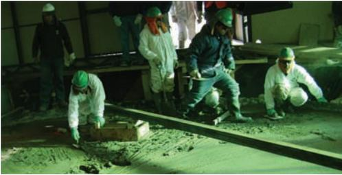
5. Workmen finishing the concrete surface. This is a final finish, since on top of this there will be additional, rather thin, layers. The uppermost thin layers of concrete are sloped to allow run-off after rain or snow. The space around the antenna station must be filled with soil. This is a more massive type station.
