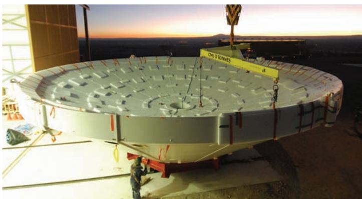
*This photo was taken at the OSF. The 1st backup structure covered with protective foams is mounted on the integration jig foreseen for panel integration, prior to be moved inside the European Antenna Consortium BUS integration building.*
