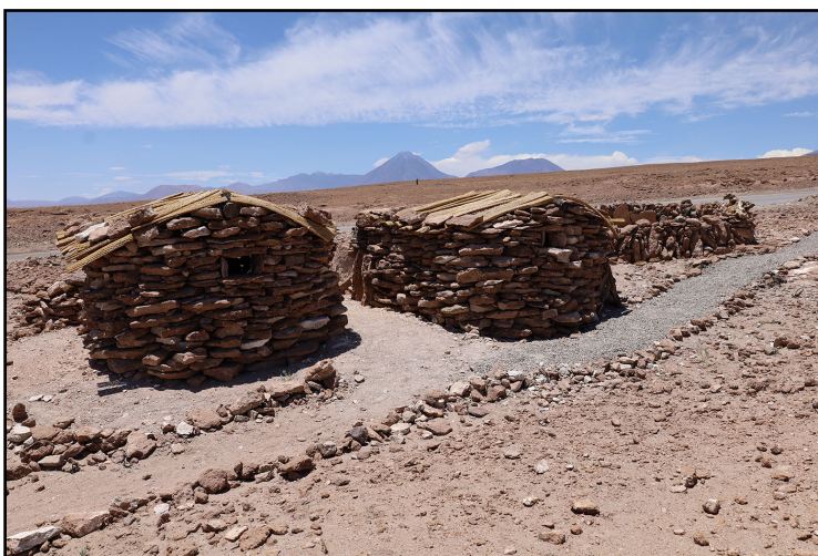
Figure 11: A partially reconstructed dwelling on the grounds of the ALMA Operations Support Facility (OSF), consisting of a kitchen/sleeping hut, corral, and "corralito" for small animals. These dwellings were in use into the 1940s by the Atacameña shepherding people who lived here. ALMA assumes responsibility for the habitat located around the observatory facilities, under archaeological advisement with San Pedro de Atacama and Chilean authorities. (Credit: G. Schieven).
