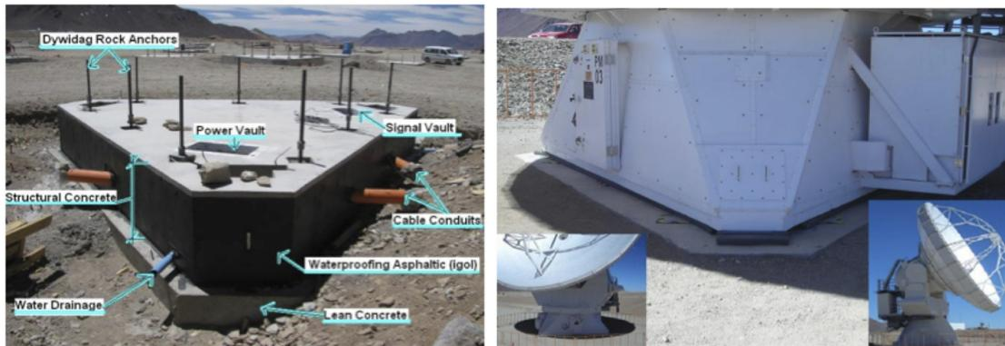
Figure A.2: Structure of an antenna pad (actual pad at the OSF) (left) and detail of antenna anchored to a pad (right).
