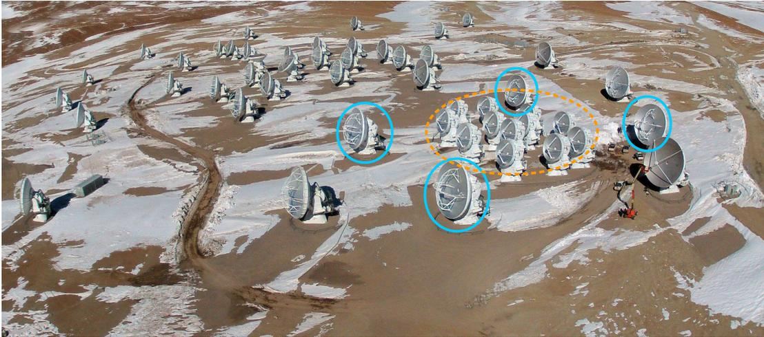
Figure 2.1: The ALMA 12-m Array in its compact configuration (left hand-side of the image). The ACA with all CM and 4 PM antennas are distributed in the right hand side of the image (circled). A few unoccupied stations can be seen, to which antennas of the 12-m Array can be moved by the transporter as the array is being reconfigured. At its most extended configuration, antenna baselines in the 12-m Array will reach a maximum extent of about 16 km.
