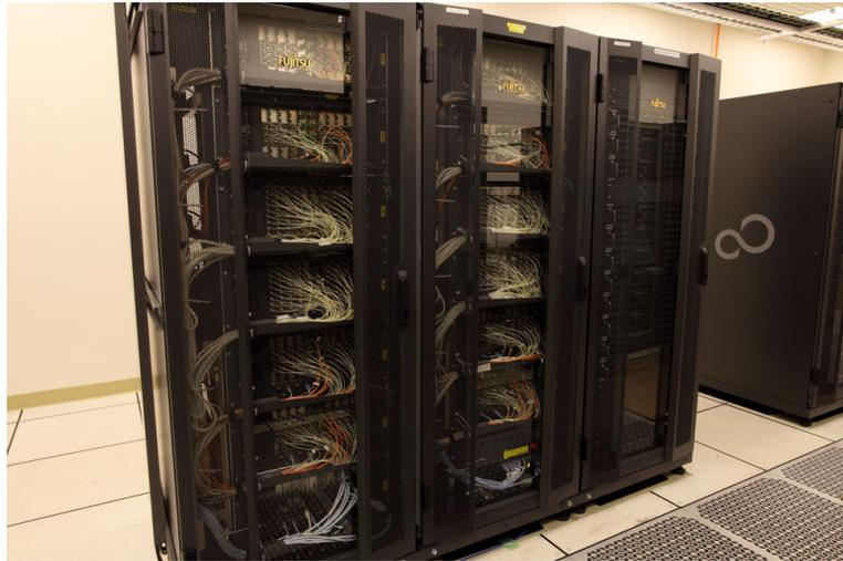
Figure 3.6: A quadrant of the ACA correlator. The left and middle racks compose a quadrant, which processes a baseband pair from sixteen antennas. The right rack is one of four computing racks, which have correlator control, post processing computers, network instruments and so on.
