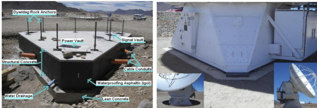
Figure A.2: Structure of an antenna pad (actual pad at the OSF) (left) and detail of antenna anchored to a pad (right).
